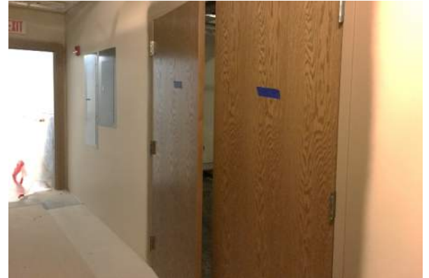
New doors and hardware being installed in the Education area.
