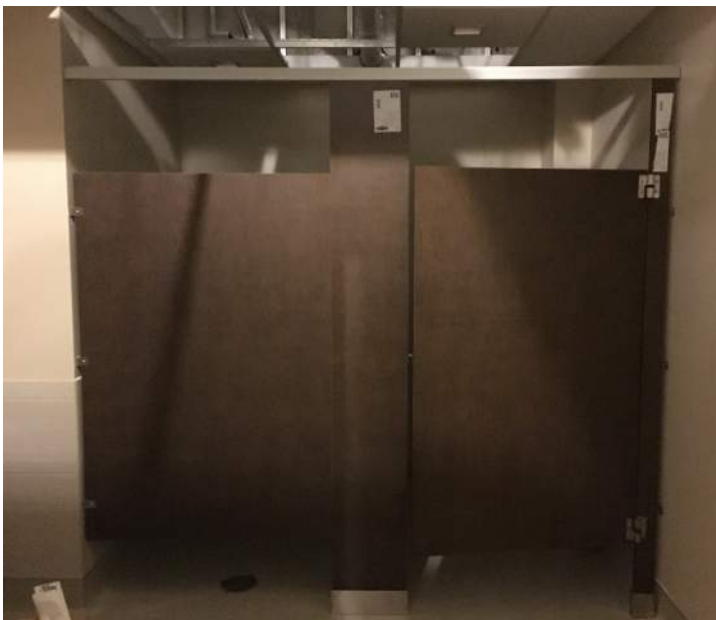
Bathroom partitions were installed in the new Education area.
